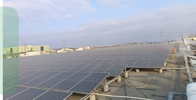
Photovoltaic power generation across all industrial parks
