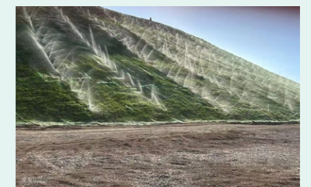
Slope spray irrigation system at the waste dump
