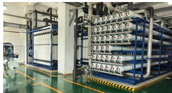
The Coal Coking and Chemical Branch carried out a project for advanced treatment and reuse of phenol-cyanide wastewater.
